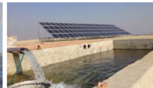
Other related water treatment uses
